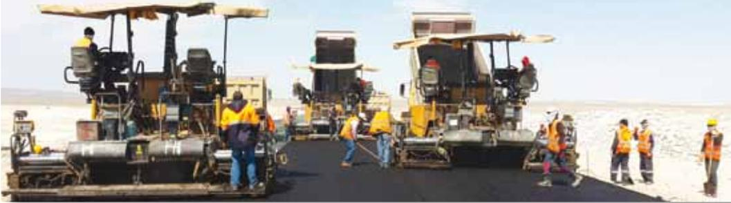
**T**he project's construction time is 30 months and mobilization was completed in 2012. A total of 114 km of road construction was completed in 2013. The project will be completed with the construction of the remaining 86 km in 2014. The contract includes earth works, culvert and drainage constructions, bridge, road sub-base, base, porous asphalt, binder and asphalt surface course works as well as vertical and horizontal road signs and markings.
