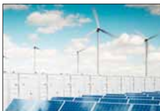
MEDAŞ Will Continue Providing High-Quality and Sustainable Power Supply with Its Power Storage Project
